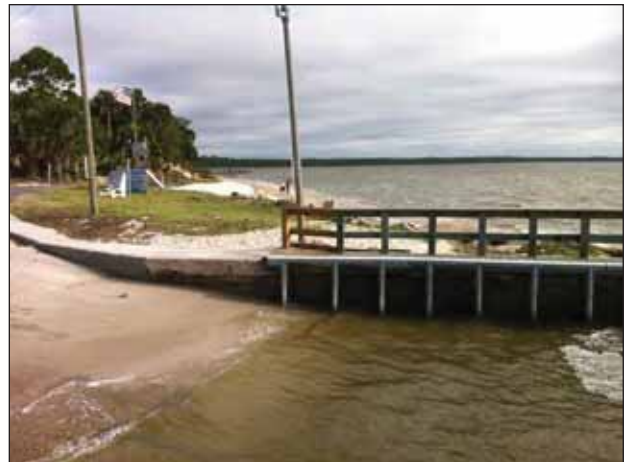
Figure 6-2B. The existing Indian Pass boat ramp.
