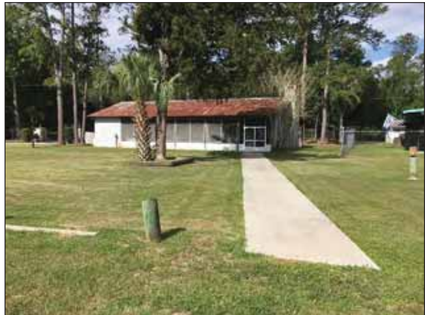
Figure 12-1C. Existing property manager's facility.
