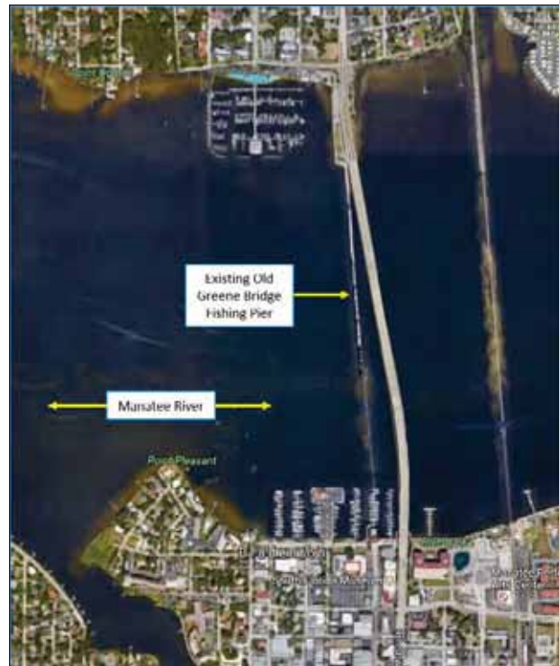
Figure 18-5B. Aerial photograph of the old bridge, immediately west of the new bridge.
