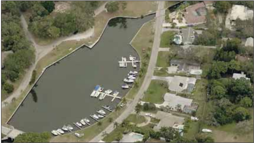
Figure 18-2B. Aerial photograph of Portosueno Park.
