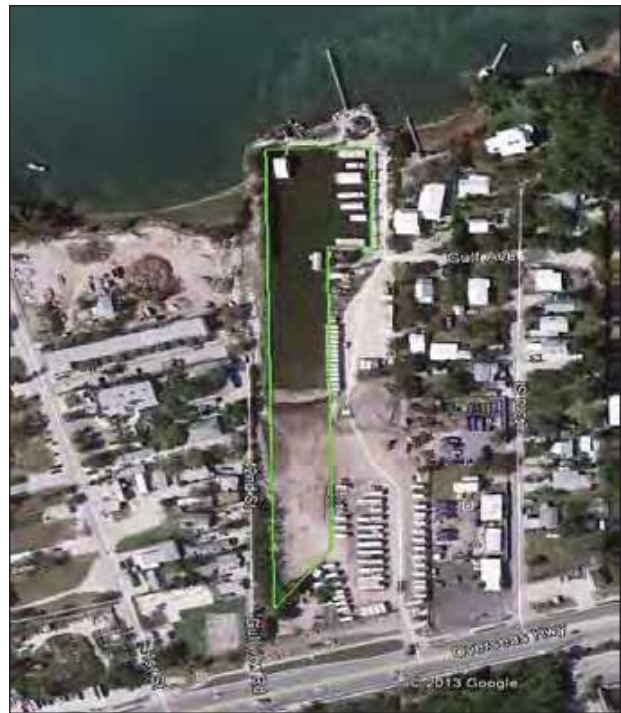
Figure 23-1C. A canal shallowing demonstration project under construction.
