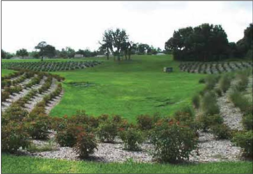
Figure 13-4B. Regional stormwater treatment facility in Citrus County.
