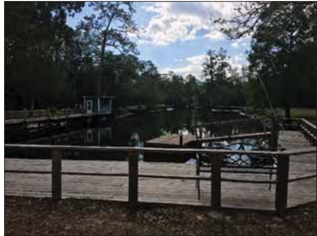
Figure 12-1B. Existing boat ramp and dock facility.
