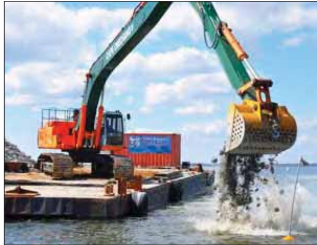
Figure 7-2C. Cultch being placed on a bay bottom from a barge for restoration (source: White 2012).
