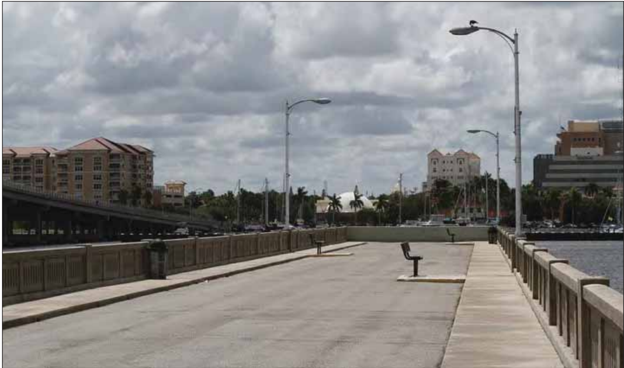
Figure 18-5C. Ground level photograph of the existing concrete fishing pier.
