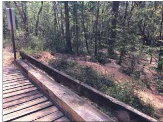
Figure 3-4D. Dorcas Road at Pond Creek Bridge with significant sedimentation next to the bridge.
